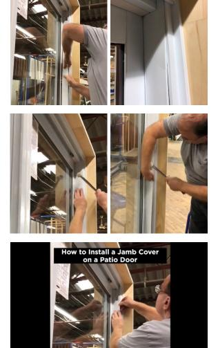
**1.** Install the top jamb pocket cover 3-4" far for the head, then slide the jamb cover up to ensure that the head end is tucked into the head-track.
