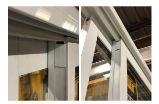
Tap the sash screw end covers into place at the top and bottom of the operable sash, as pictured.
